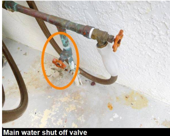
Main water shut off valve
