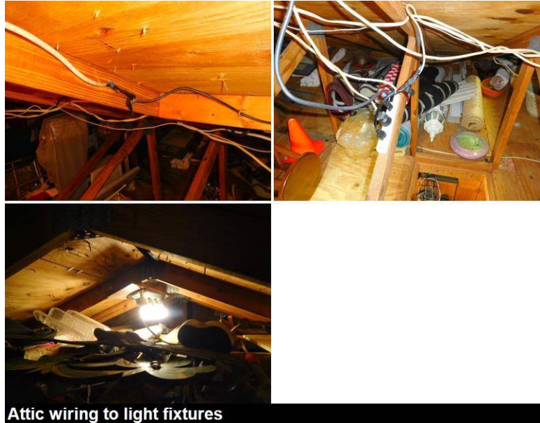
Attic wiring to light fixtures
