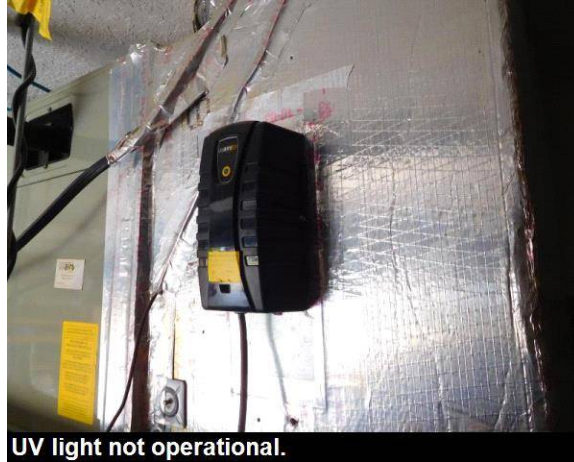
UV light not operational.
