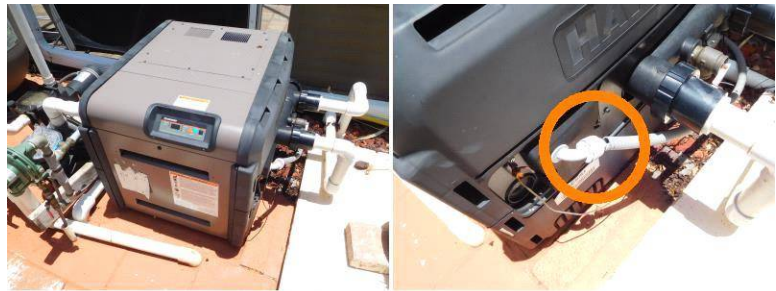
Heater not operational / Loose conduit
