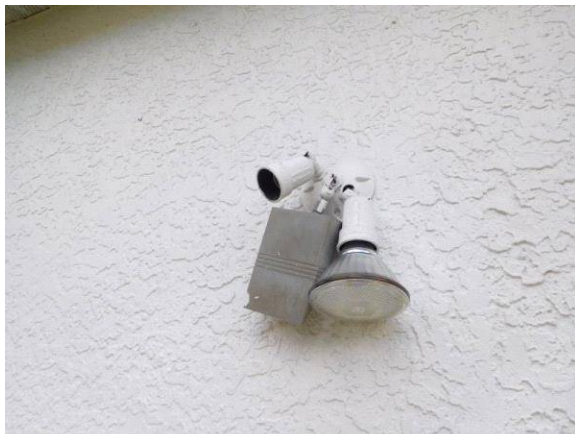
Damaged flood light fixture
