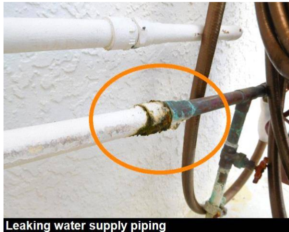
Leaking water supply piping
