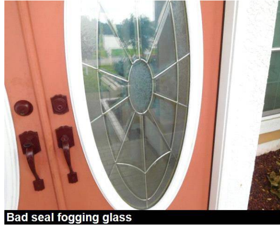
Bad seal fogging glass
