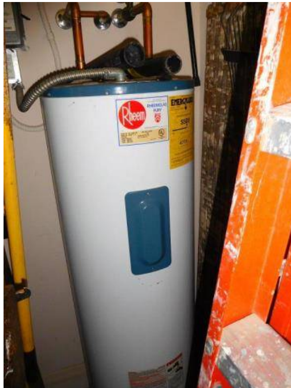
Age of Water Heater unit is, 8 years old. Electric, 4500 watts, Rheem.
