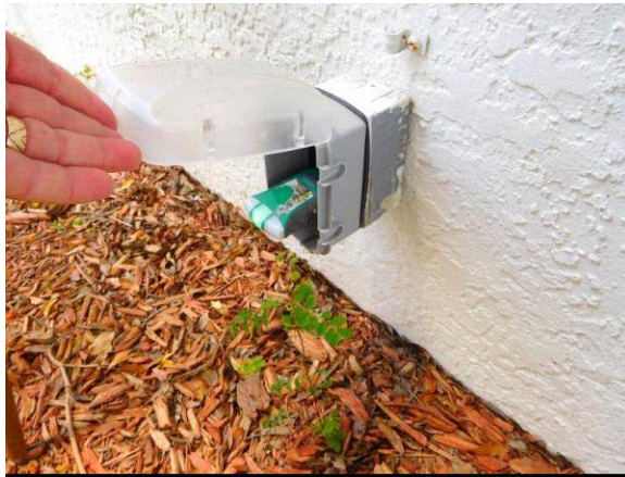
Typical missing GFCI protective outlet
