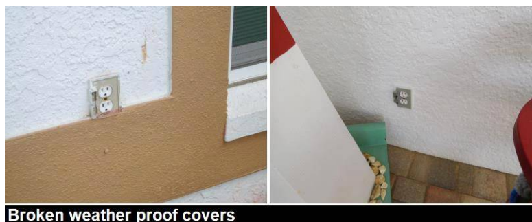
Broken weather proof covers
