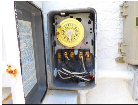
Missing protective cover
