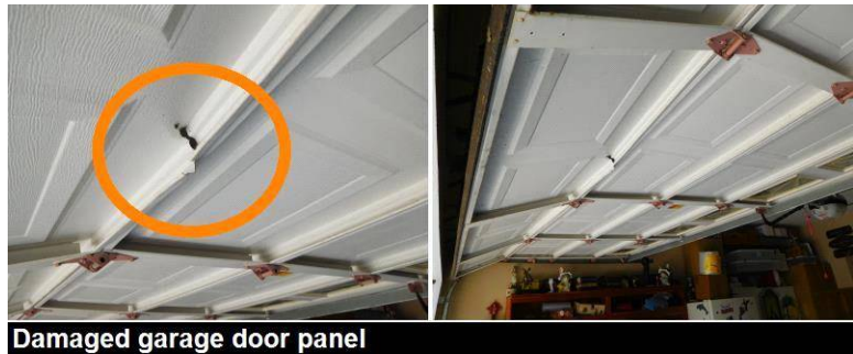
Damaged garage door panel
